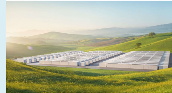
129 MWh stabilisation station within an Australian wind-generator field Hornsedale Power Reserve . Tesla 2018
