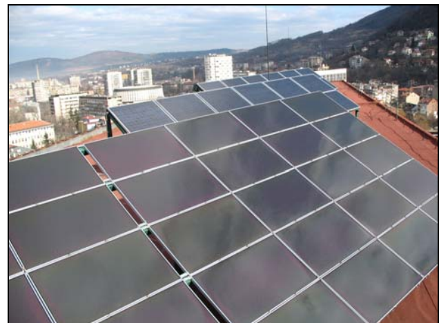
Figure 1. Grid connected photovoltaic power plant on the roof of the Rectorate of Technical University of Gabrovo
