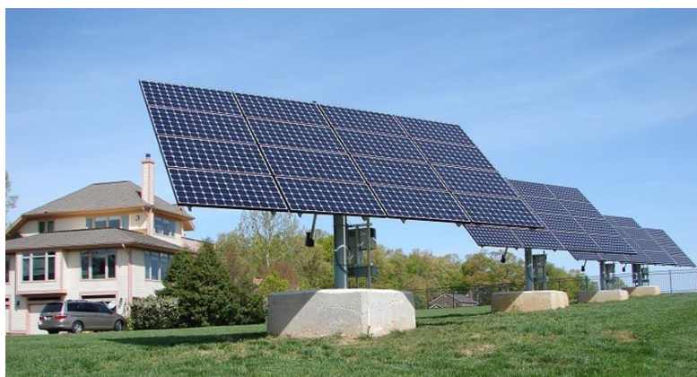
Figure 3. One-axis tracking PV solar power plant [9]
