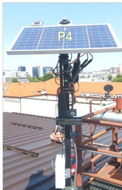
Figure 7. Experimental dual-axis tracking PV system with 50 W polycrystalline silicon solar module
