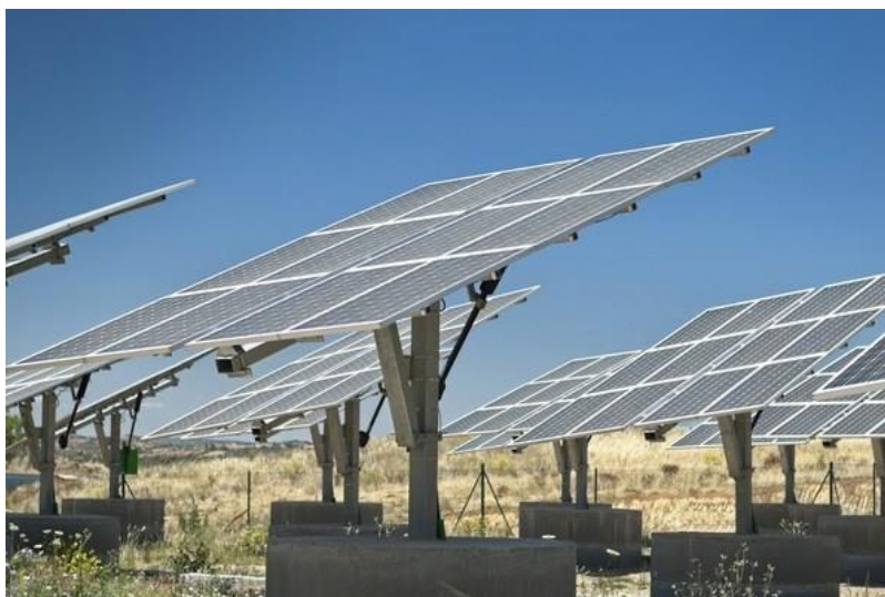
Figure 4. Dual-axis tracking PV solar power plant [10]
