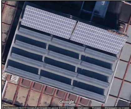
Figure 10. Satellite photo (Google) of 132 kWp roof-mounted solar power plant in the industrial enterprise ZITA. [23]
