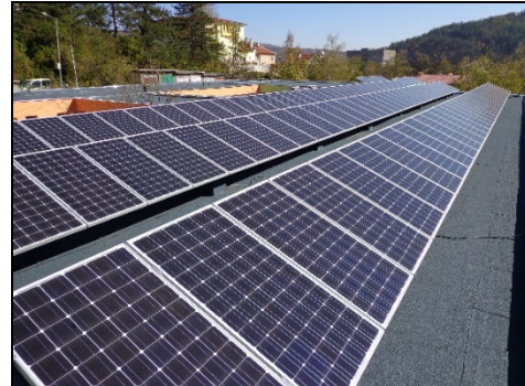
Figure 11. 23.76 kWp grid connected PV system on the roof of the kindergarten „First June“ in Gabrovo
