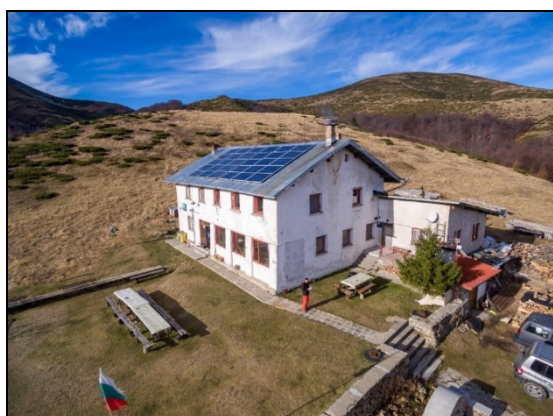
Figure 18. Autonomous PV system for power supply of high-altitude mountain information center Tazha hut in National Park „Central Balkan“ [30]
